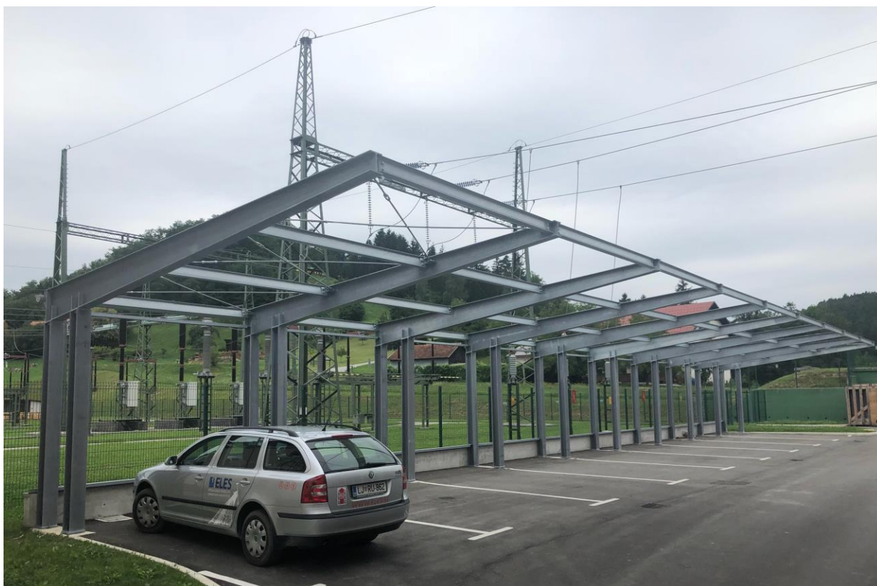
Figure 13: Steel Canopy for Vehicles during construction
