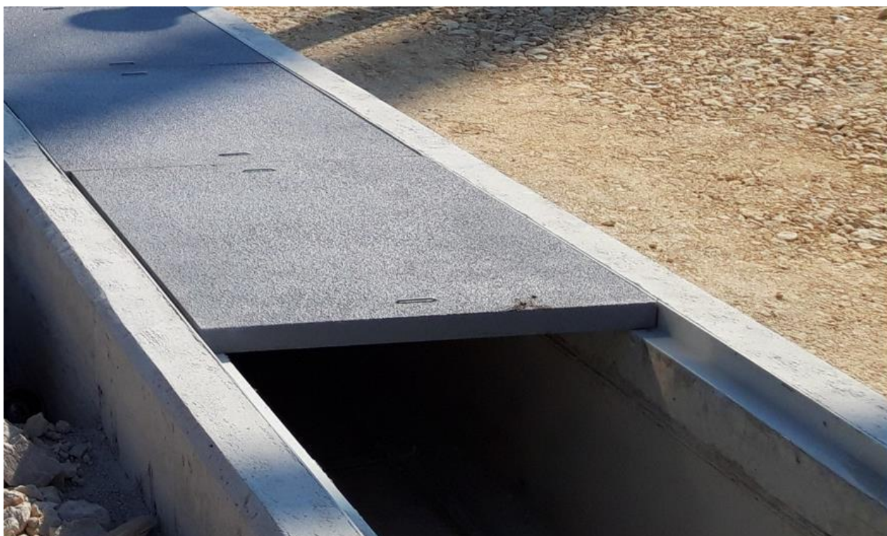
Figure 22: Reinforced concrete channels with covers made of reinforced polyester (designed for pedestrian-accessible areas)
