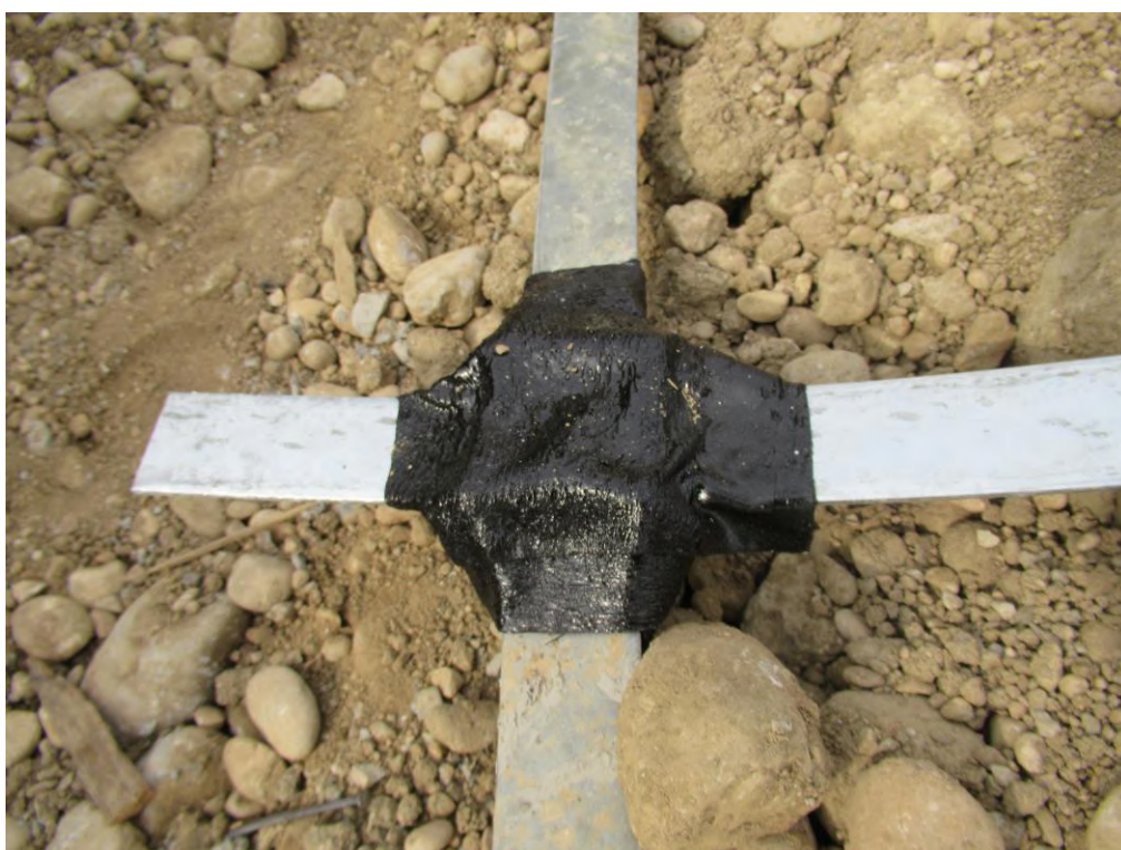
Figure 3.2: An example of a cross clamp protected with a Corodal tape
