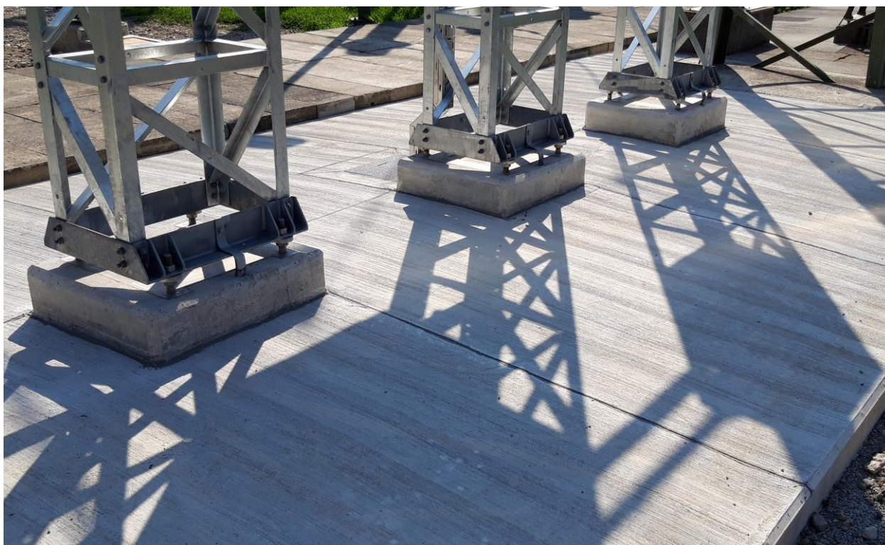
Figure 24: Reinforced concrete equipment service and access platform
