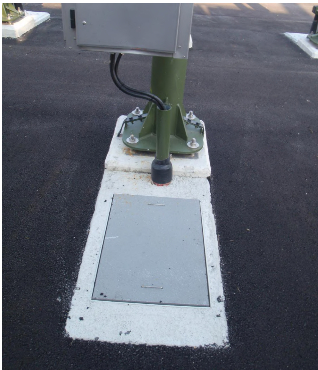
Figure 17: Typical solution for routing equipment wiring into a cable trench alongside the foundation of the equipment support structure
