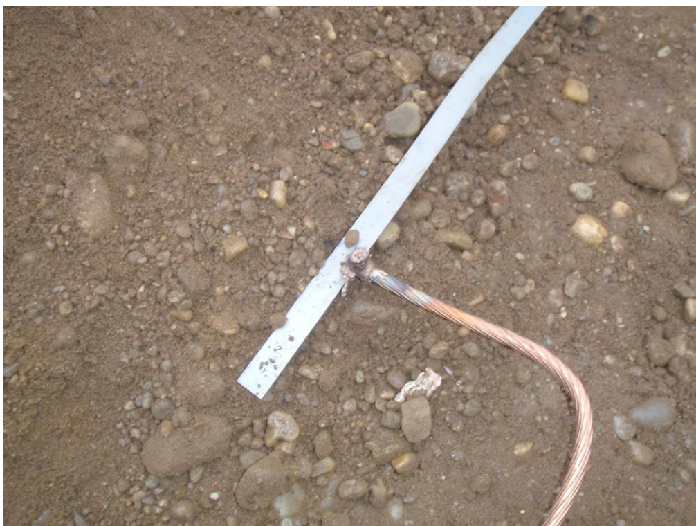
Figure 3.1: Example of an exothermic connection between a FeZn 40x4 mm and a copper earthing rod
