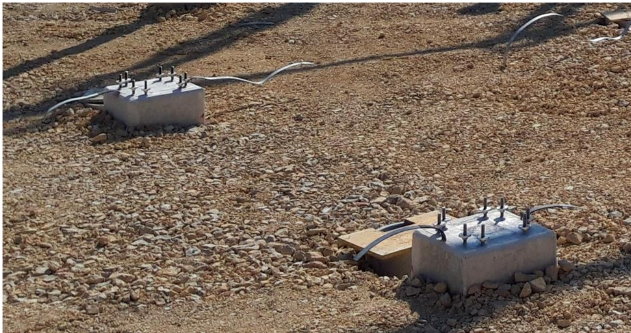
Figure 16: Pre-installed Anchors in Foundations for Equipment Supports
