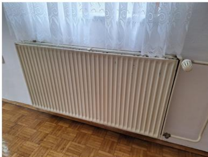
Slika 31: Panelni radiator s termostatskim ventilom in termostatsko glavo
