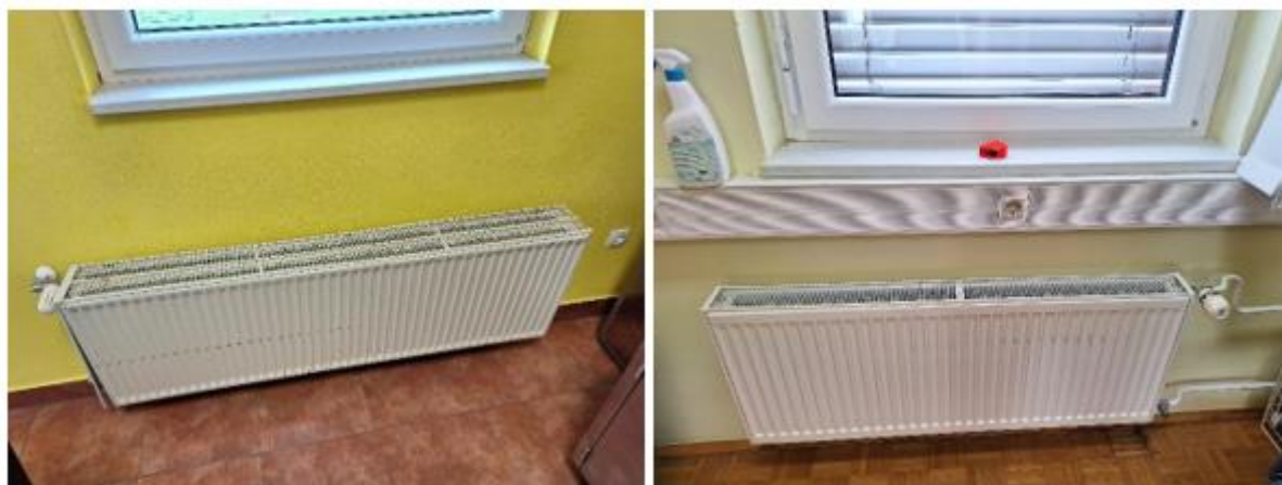
Slika 18: Panelni radiator s termostatskim ventilom in termostatsko glavo
